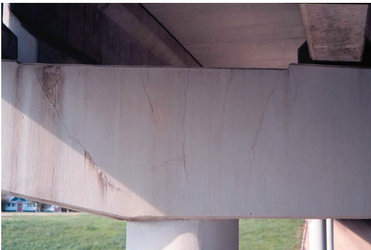
Figure 1. Cracking in TxDOT Bent Cap
