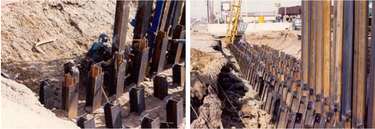
Figure 43 – Example of Bridge Foundation Using Steel H-Piles
