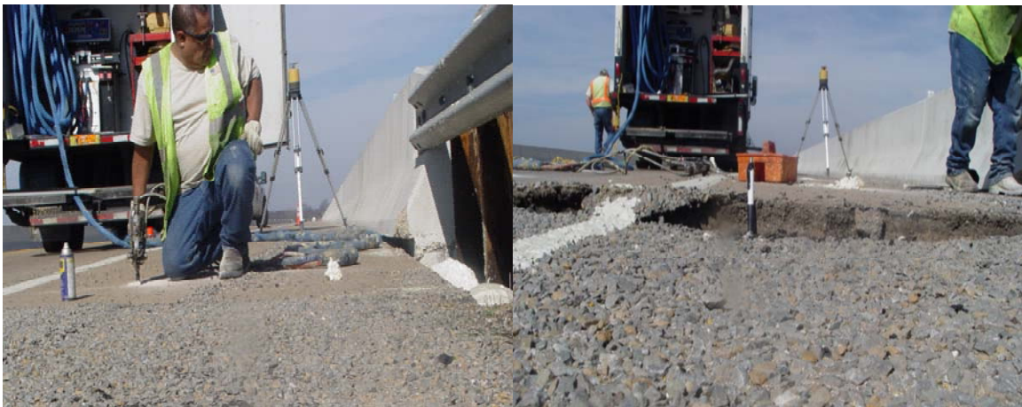
Figure 67 – Position of Approach Slab during and after the Urethane Injection Process
