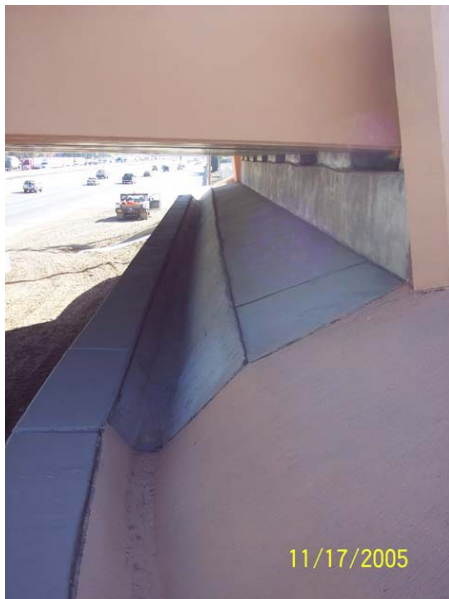
Figure 59 – Concrete Slope Protection with Drainage Gutter and Drainage Channel (Lenke, 2006)
