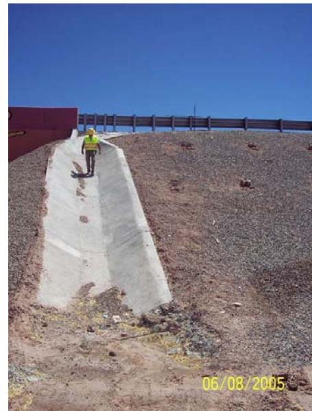
Figure 59 – Concrete Slope Protection with Drainage Gutter and Drainage Channel (Lenke, 2006)
