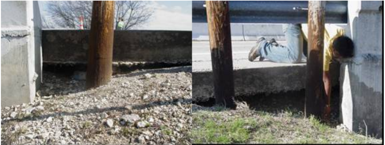
Figure 66 – Schematic of the Approach Slab with Developed Void under the Bridge at FM 1947 Hill County, Texas
