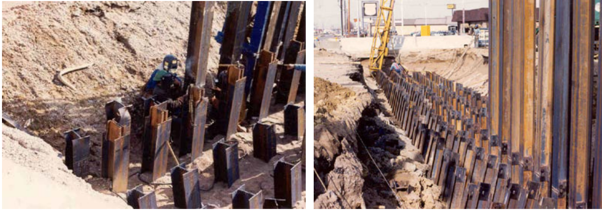
Figure 2.43. Example of Bridge Foundation Using Steel H-Piles.
