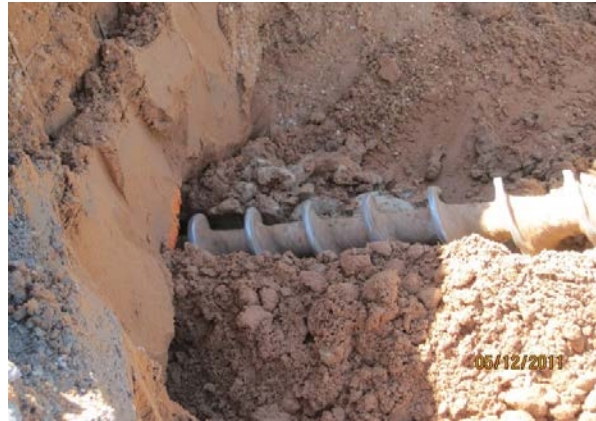
Figure 9.17. Drilling of Holes to Place the Soil Nails.
