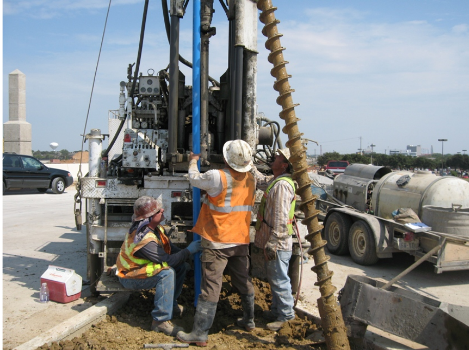
Figure 6.16. The Casing Installation after Reaching the Required Drilling Depth.
