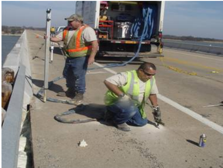
Figure 9.9. Taking Elevations during the Injection Process to Check for Extra Injection.
