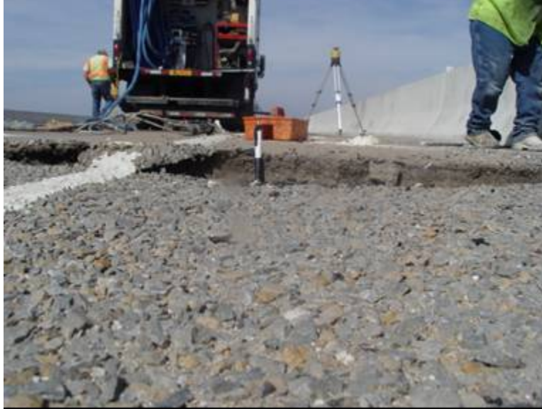
Figure 9.10. Pavement Differential of the Lifted Approach Slab during the Injection Process.
