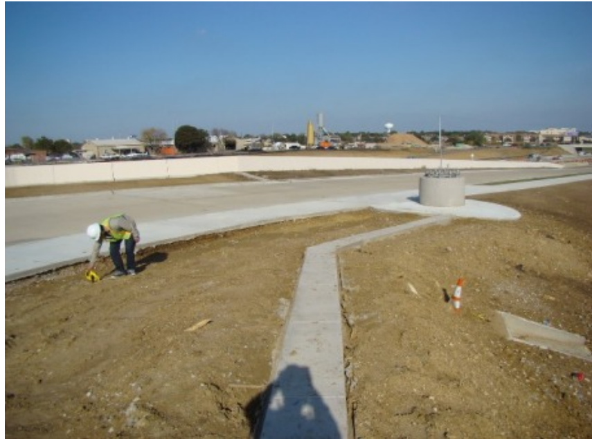
Figure 7.4. The Location of the Broken Casing.
