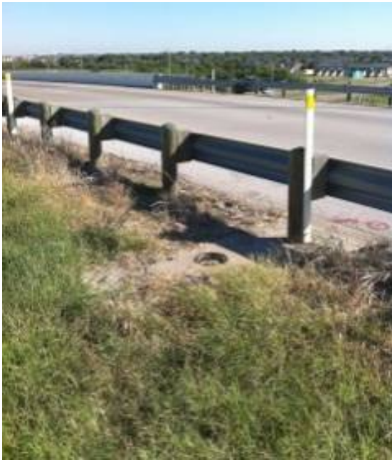
Figure 7.26. Inclinometer V3 Platform close to the Highway Shoulder.
