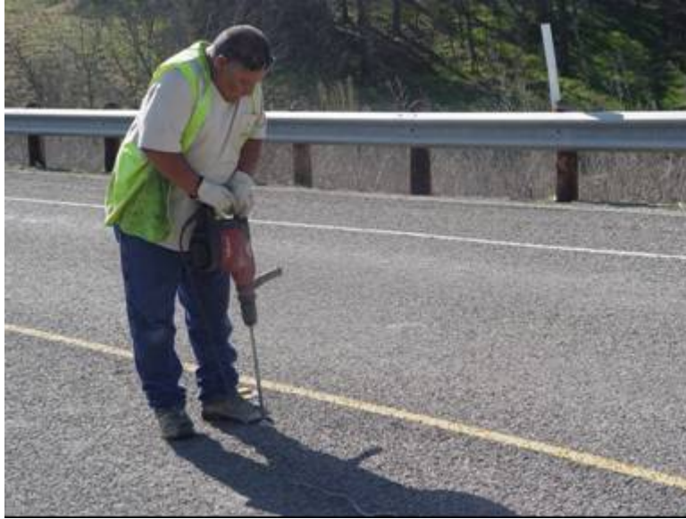
Figure 9.6. Drilling Holes into the Approach Slab.
