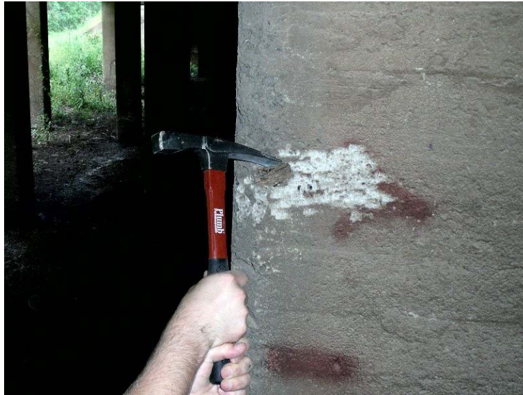
Figure 4. Hammer Test of Concrete Condition.
