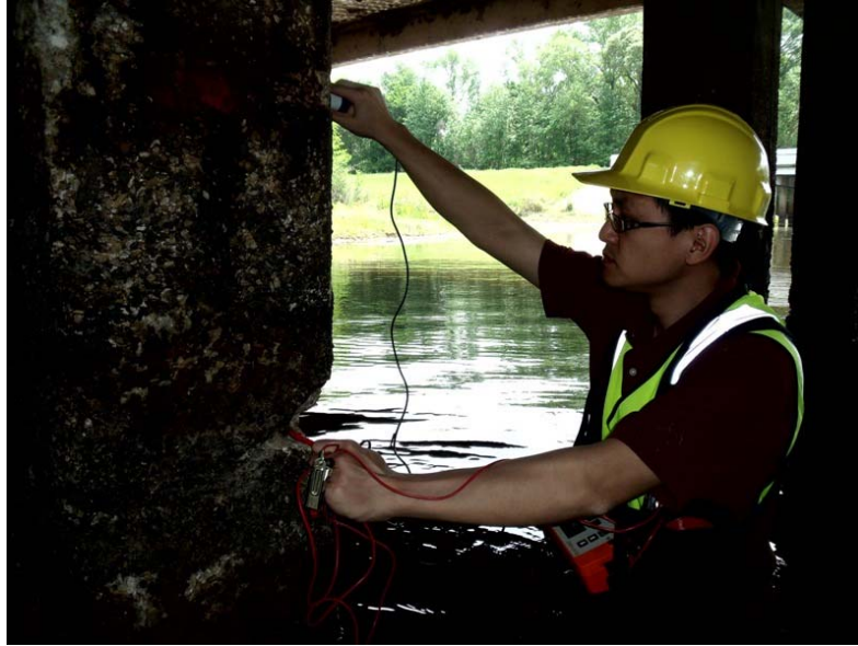
Figure 8. Half-Cell Corrosion Potential Test.
