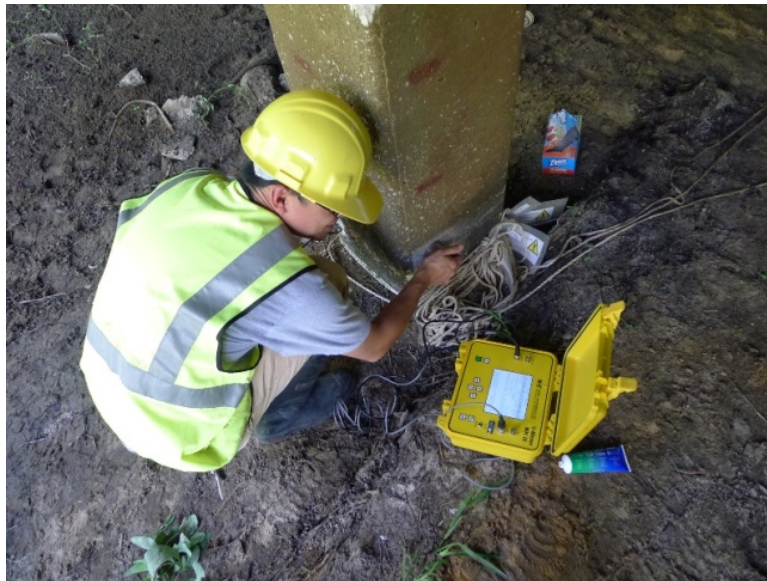
Figure 6 Ultrasonic Pulse Velocity (UPV) Test.
