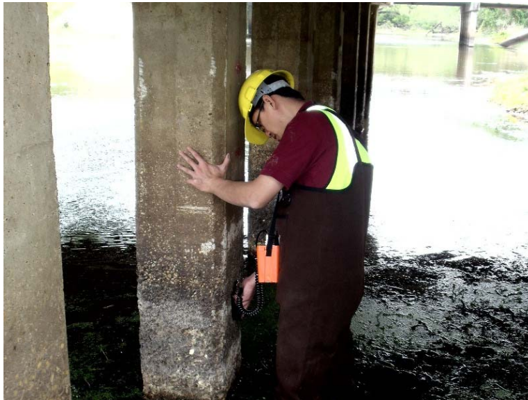
Figure 7. Covermeter (Rebar Locator) Test.
