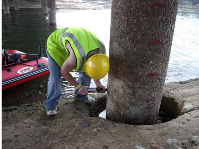
Figure 5. Schmidt Rebound Hammer Test.
