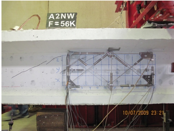
(a) First shear crack at 56 kips
