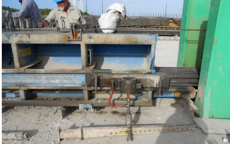
Fig. 6.16 Bed Vibrator Attached to Steel Forms
