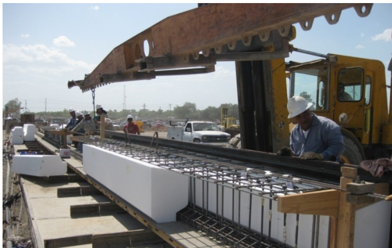
Fig. 3.17 Installation of Styro-Foam Forms
