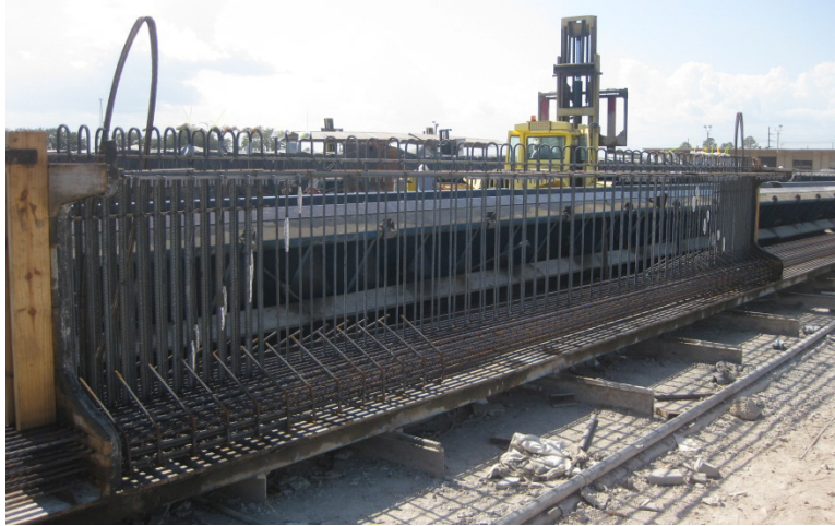
Fig. 6.13 Reinforcement Cage for a Typical Girder
