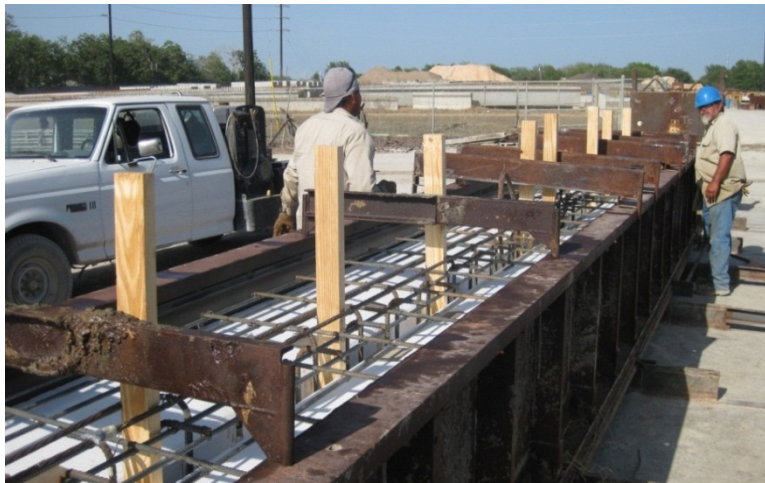
Fig. 3.18 Set-up of Steel Side Forms for Girders
