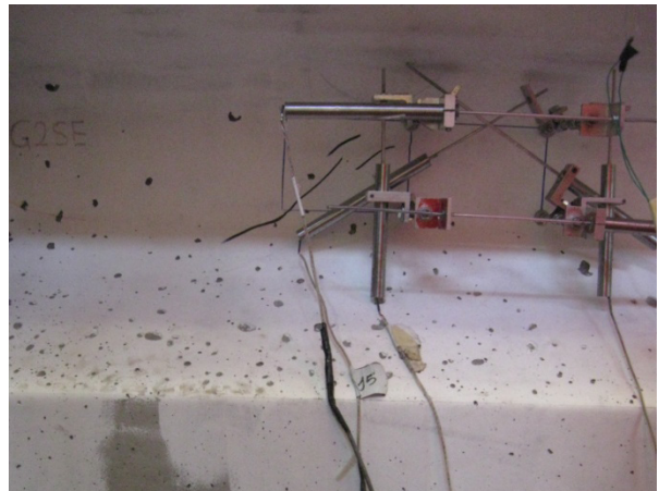
(b) First shear crack at 213 kips
