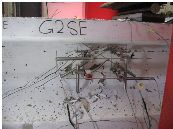
(f) Shear failure at 524.64 kips
