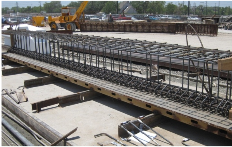
Fig. 3.15 Reinforcement Cage for a Typical Girder
