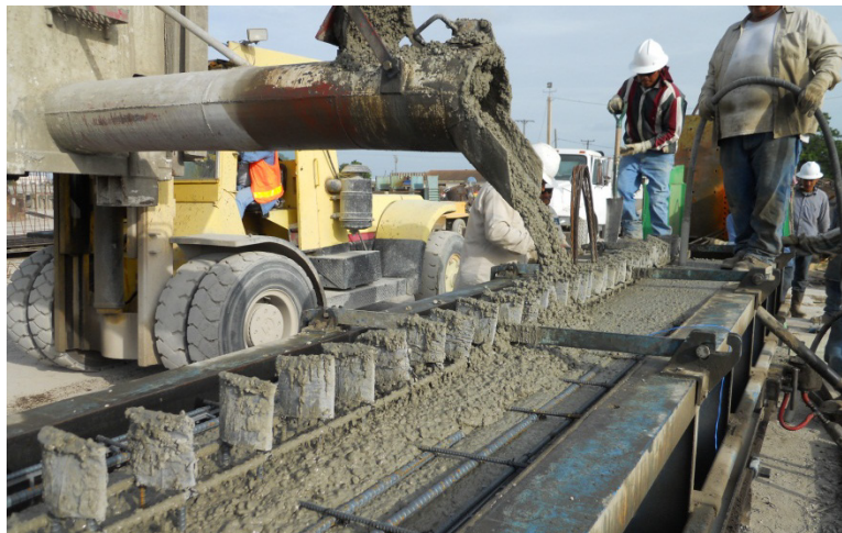
Fig. 6.15 Concrete Placement Using a Hopper
