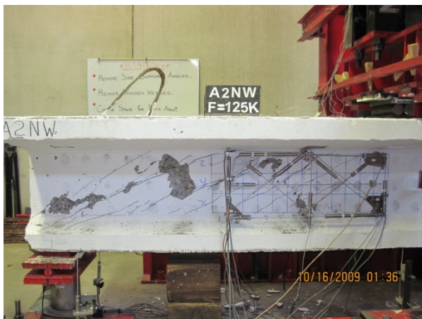
(e) Shear failure at 125.60 kips
