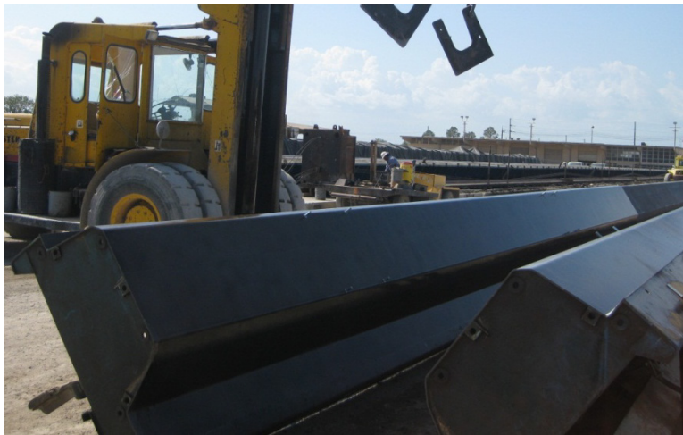
Fig. 6.14 Coupling Nuts Fixed in Steel Forms
