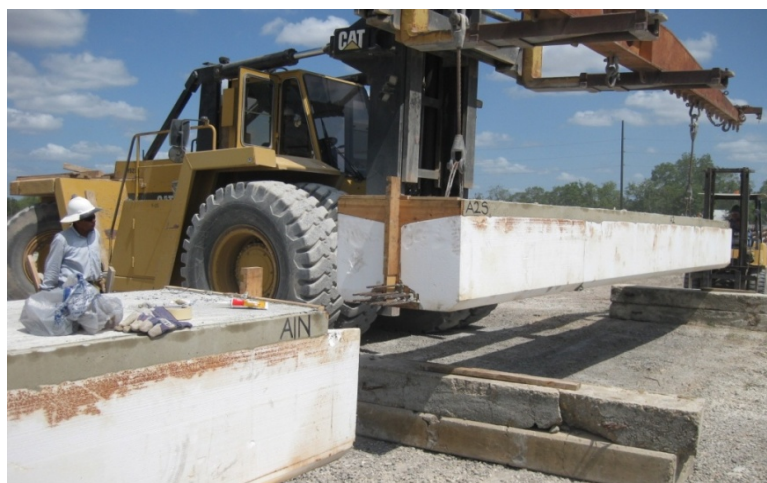
Fig. 3.20 Removing Styro-Foam Forms from the Girders
