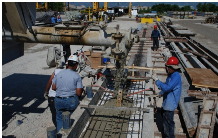
Fig. 3.19 Concrete Placement Using a Hopper
