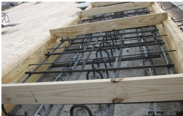
Fig. 6.17 Reinforcement Cage for Top Slab
