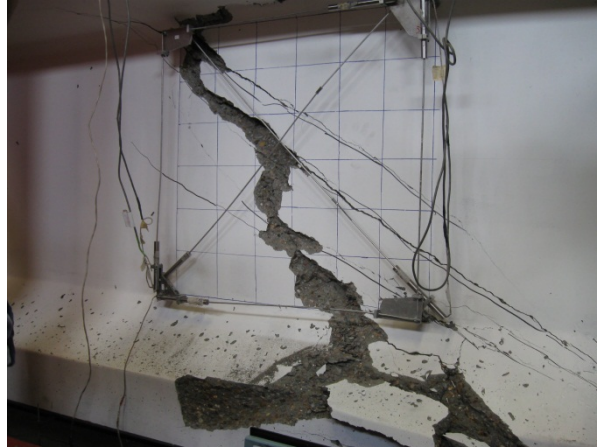
(c) Shear failure at 756.42 kips
