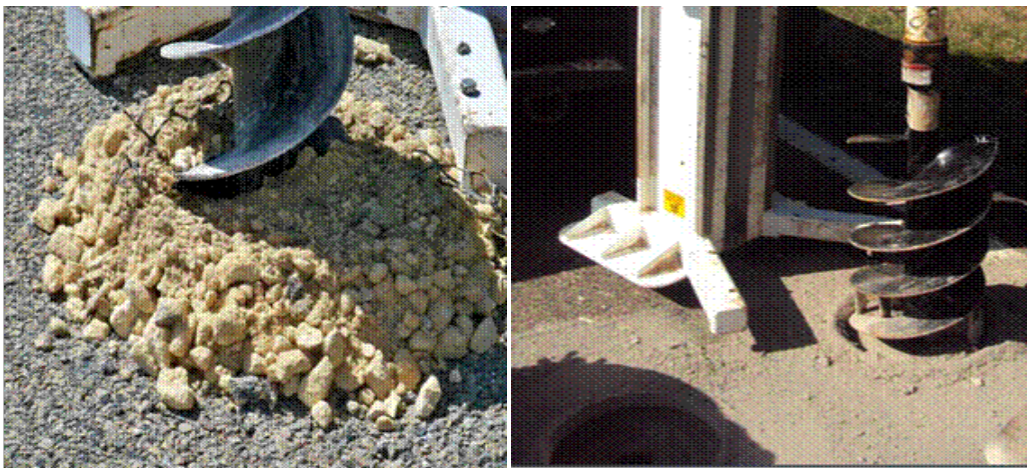
Figure 4.2. Material Sampling using Auger.
