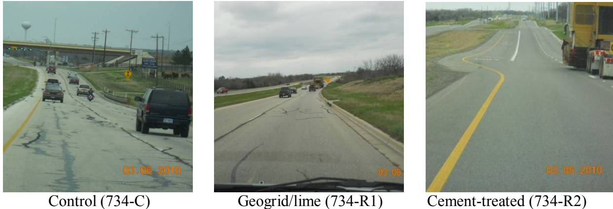
Figure 4.14. FM 734 Test Sections Surface Conditions.
