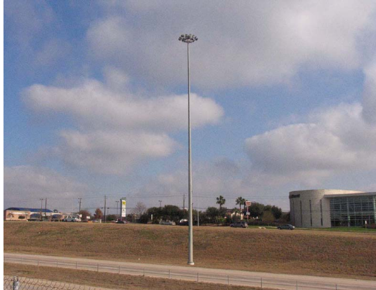
Figure 1. High Mast Illumination Pole (Rios, 2007).
