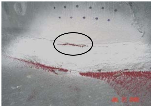
(c) Lack of fusion revealed by MPT (1/64" removed at weld toe)
