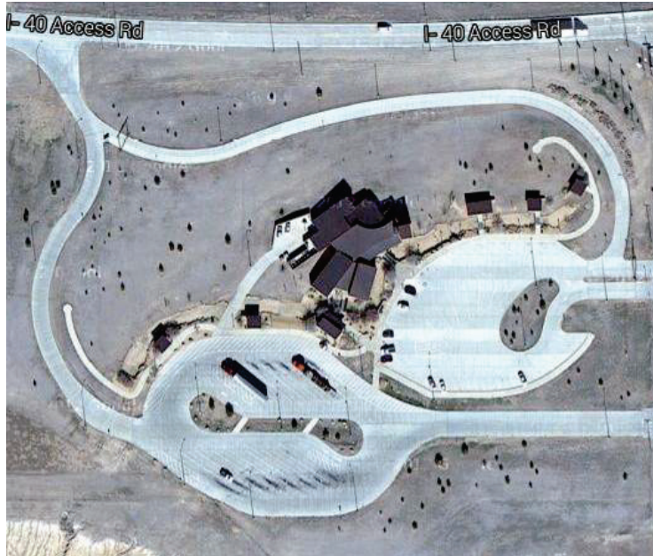
Figure 3-8. Aerial View of the Amarillo Travel Information Center.
