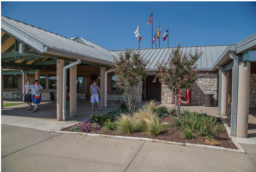
Figure 3-12. Main Entrance to the Gainesville Travel Information Center.
