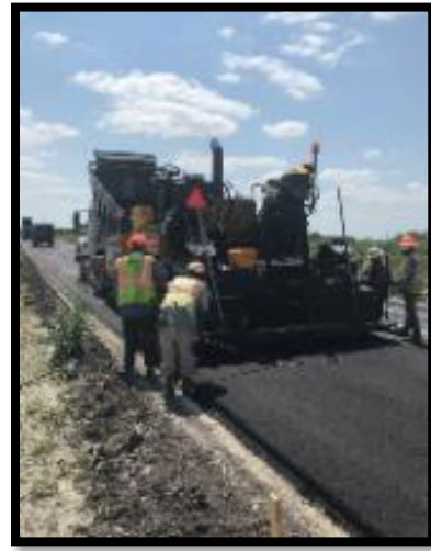
(b) Type-D mix placement
