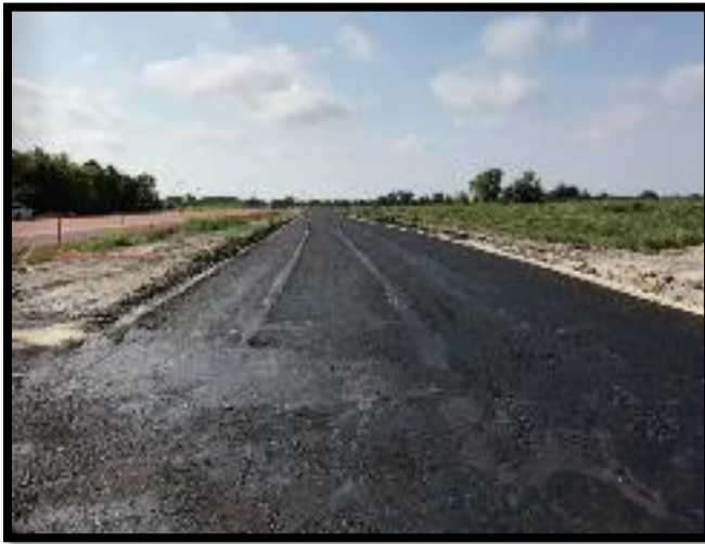
(a) Prime coat applied
