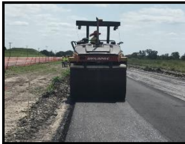
(c) Compaction with CMS system
