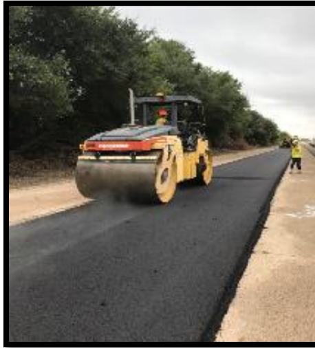
(c) Compaction with CMS system
