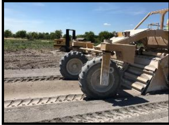
(b) Pulverization and mix
