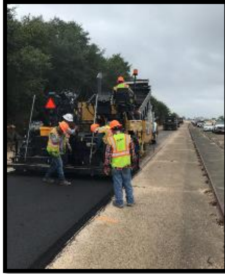
(b) Type-D mix placement
