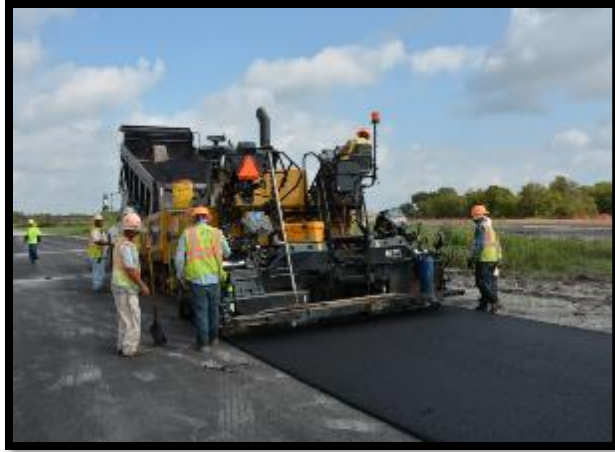
(a) Flexible pavement section
