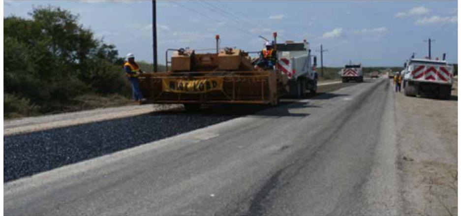
Surface treatments are seal coats/chip seals applied to the top of primed flexible base course. Surface treatments are a pavement surfacing layer constructed by the spray application of an asphalt binder followed by the distribution and rolling of a nearly one sized aggregate. Single or multiple layers of the combination of sprayed asphalt binder and distributed and rolled aggregate are widely used in Texas.
