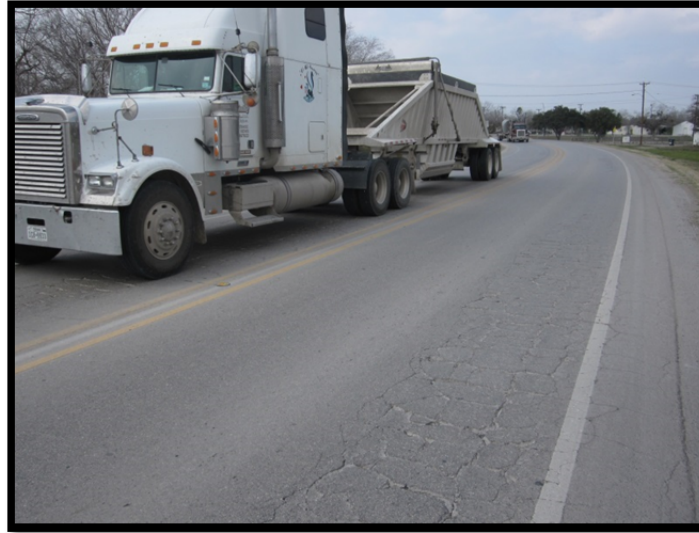
Figure 2. Alligator Cracking.
