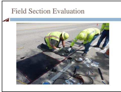
Two layers of the UT mixtures were applied on square sections of 3 ft x 3 ft. The mixture was applied manually and spread very fast before it dried up. Each patch was divided into small 4 equal bays to apply the material. After about two hours of total curing, the DFT and CTM tests were performed.
