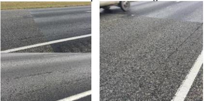
The slide contains two images showing the road surface after 18 months. The left image shows a road with a white line, and the right image is a close-up showing significant raveling and wear in the wheel paths.
