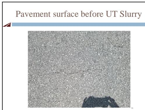
This photo shows a HMAC pavement in Beaumont prior to application of the UT slurry seal (in 2017).
