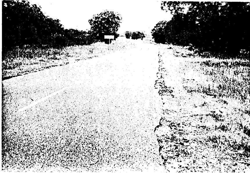
Figure 1. Expanded shale coverstone after three years of service.
