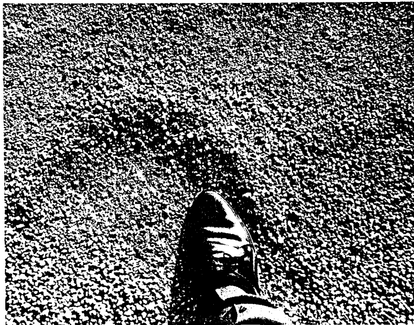
Figure 9. Skin patches made using aggregate of the same color and texture would improve the appearance of this road.
