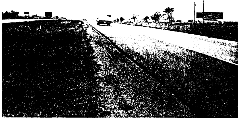
Figure 13. Section to experimental hot-mix utilizing lightweight aggregate for the inside lane. Viewed after 6 months of service. Traffic: 24,000 vpd (both directions).
