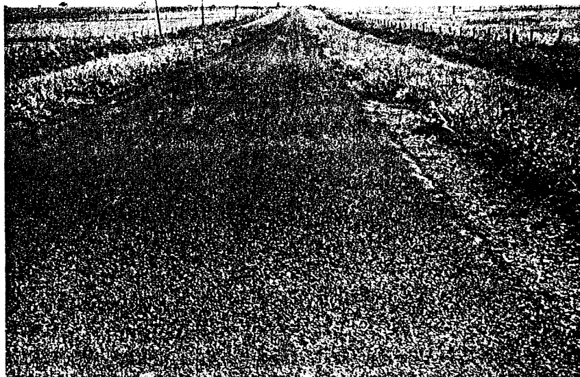
Figure 8. Low traffic volume facility utilizes lightweight synthetic aggregate as coverstone.
