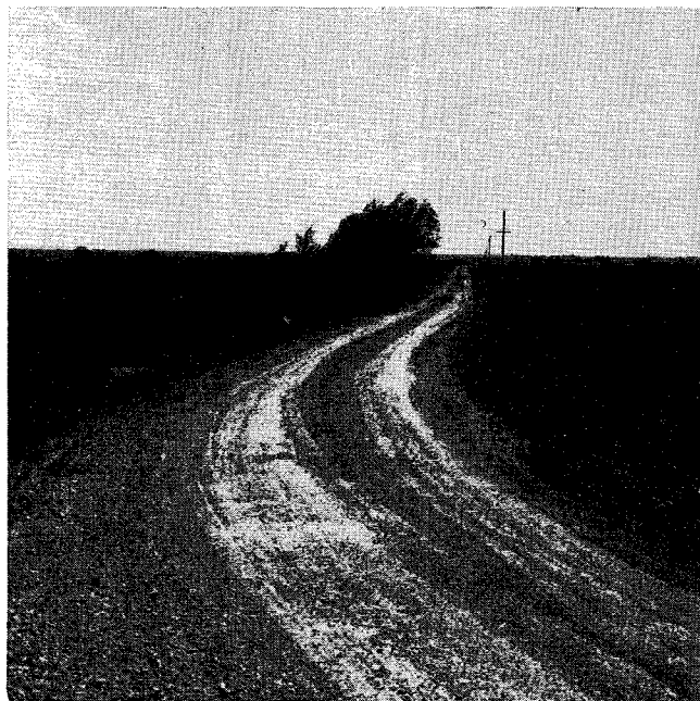
A county-maintained gravel road.
