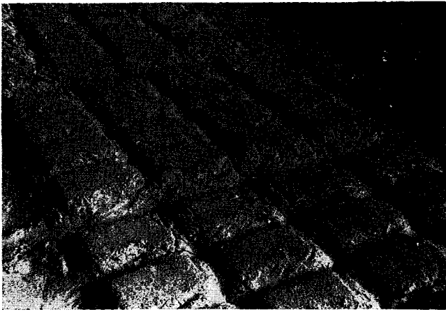
Figure 32. Inadequate protection of blocks during curing schedule may result in a loss such as occurred here after a rainstorm.
