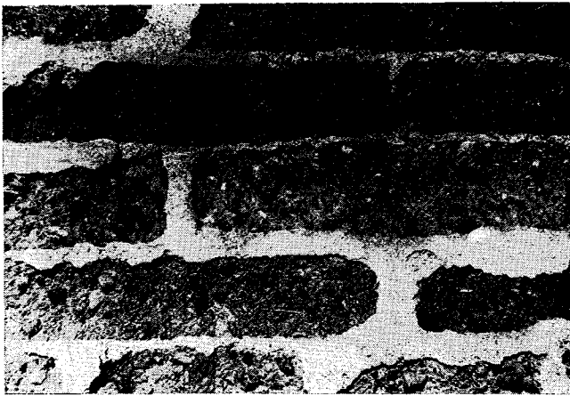
Figure 6. Close-up view of Ft. Davis, Texas, adobe wall demonstrates large aggregate in the adobe blocks.
