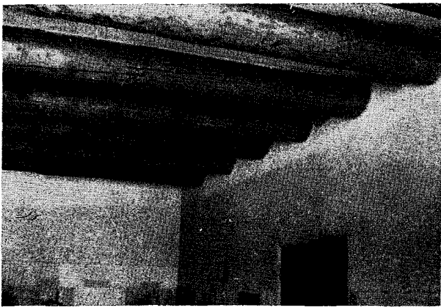
Figure 27. The large and small ends of the ceiling timbers (vigas) are alternated to provide a balanced appearance.
