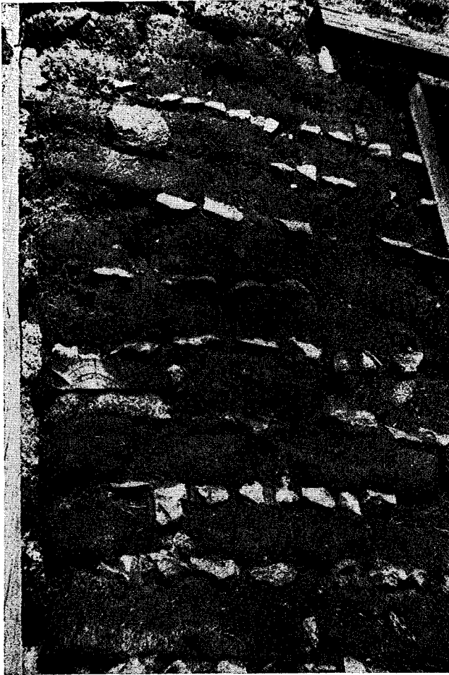
Figure 10. The mechanical bond of plaster to the adobe wall was enhanced by the early builders of Ft. Davis, Texas, by inserting rock chips in the fresh mortar.
