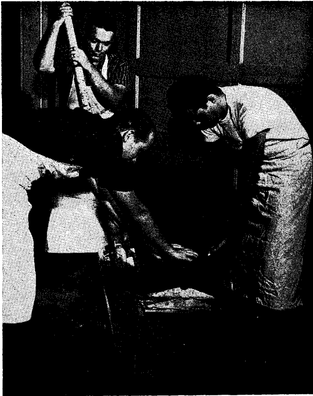
a. Charging mold box with soil mix.
