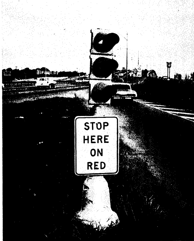
RAMP CONTROL SIGNAL
