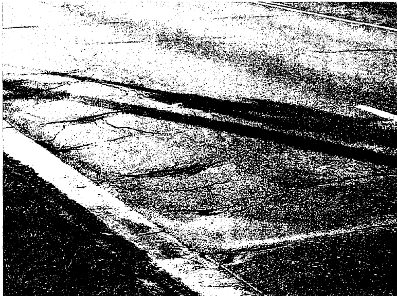
Potholes, rutting, narrow lane widths typical on Harrisburg. May contribute to side-swipe crashes.
