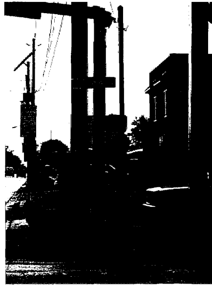
Pedestrian signal head obscured by pole from some angles
