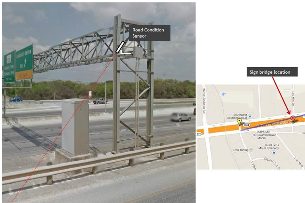
Figure E-14. San Antonio—Road Condition Sensor Installation, Roadside View.
