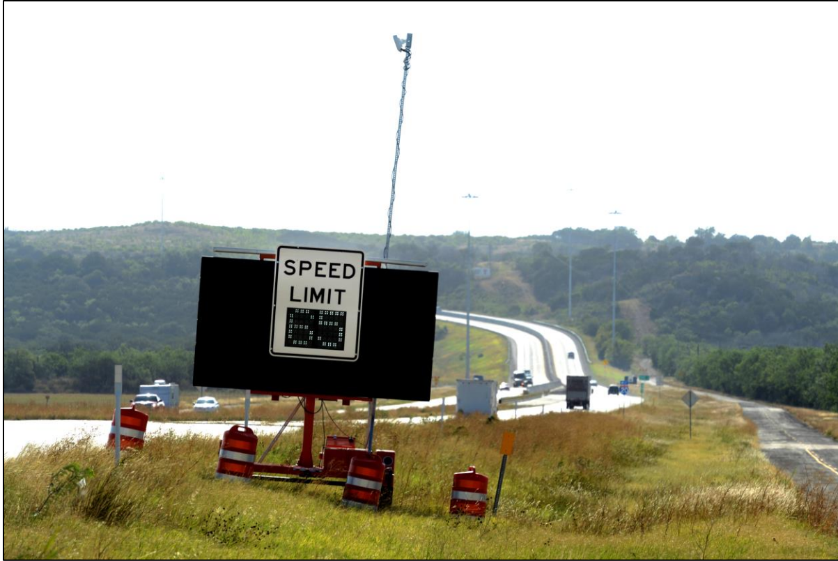
Figure 3. VSL Sign Installation, Ranger Hill, Eastland County.
