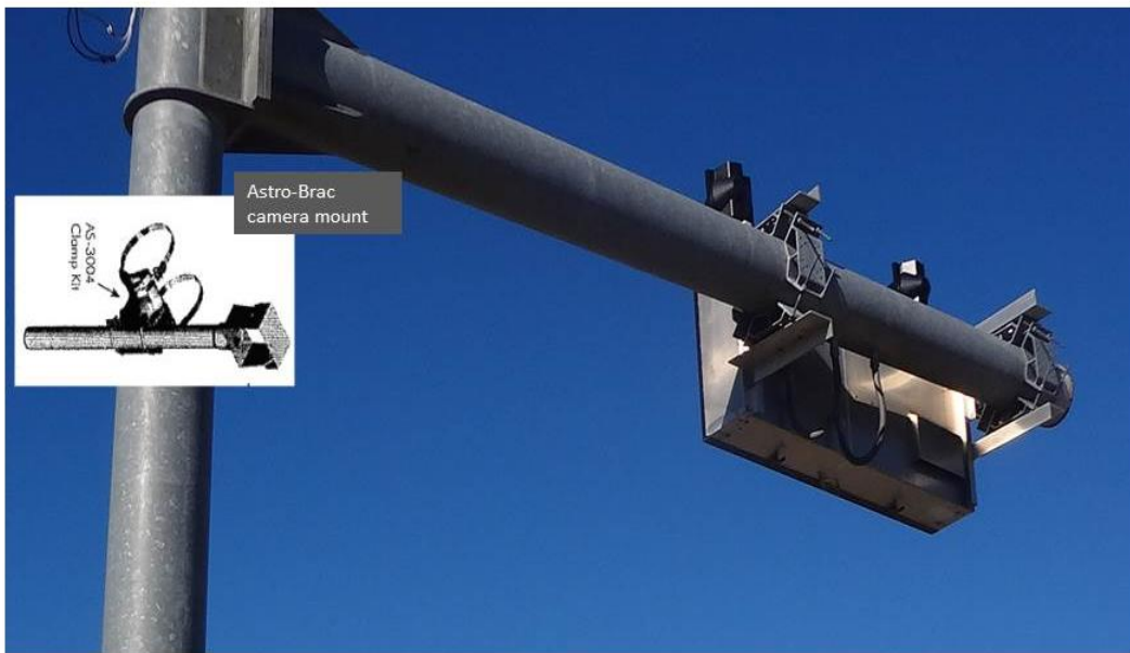
Figure E-13. San Antonio—Road Condition Sensor Installation, Closeup.
