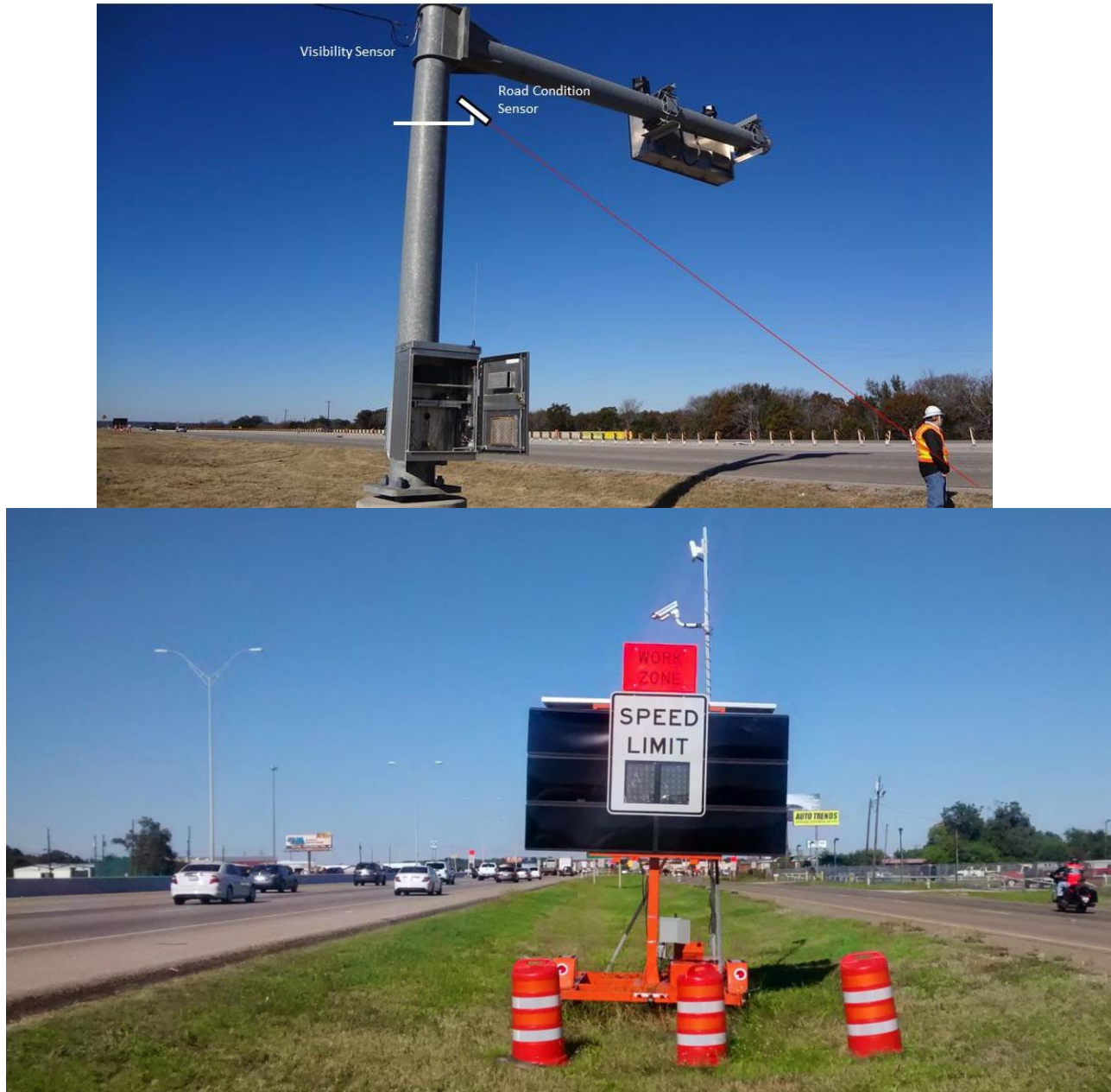
Figure E-16. Ranger Hill, Eastland County (Top) and San Antonio (Bottom)—Road Condition Sensor Installation, Roadside View.
