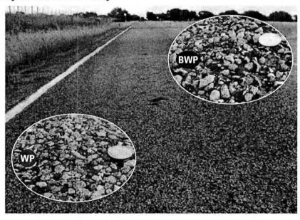
Figure 6. Lane with Slight Wheel Path Color Difference.
