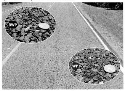
Figure 7. Lane with No Wheel Path Color Difference.
