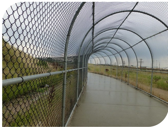
Figure 5.3. Chain link fence tunnel over bicycle trail in Cheyenne, Wyoming ( http://steveandgeorgia.net/Weblog/?p=1460 ).
