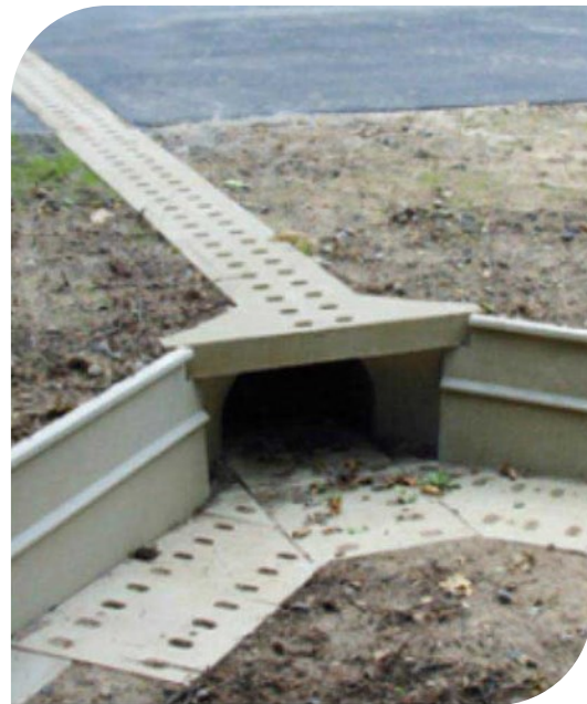
Figure 3.8. Amphibian/reptile tunnel of multiple prefabricated polymer concrete units (ca. 1 x 0.7 m, w x h) (Legacy Habitat Management Limited 2019)
