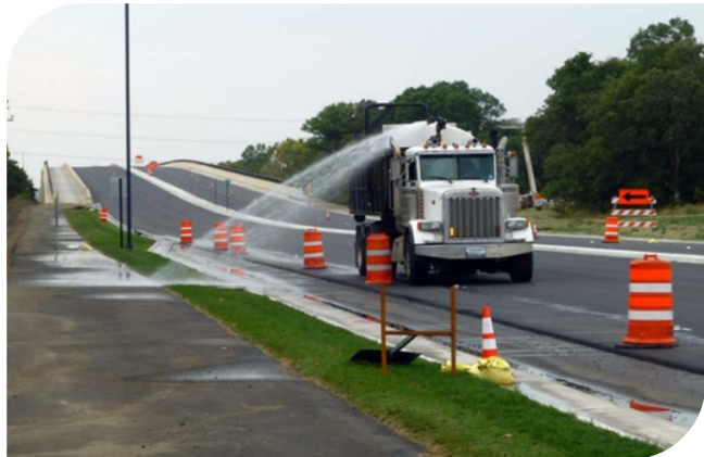
Figure 6.14. MnDOT roadside watering of turf plantings (UNM-CTS 2017)
