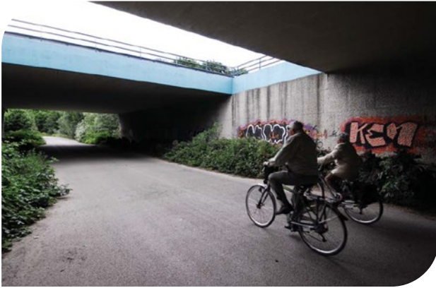
Figure 3.6. Multi-use underpass box culvert (ca. 1.5 x 1.5 m, w x h) for ocelots along FM 106 at Ted Hunt Road, Texas (USDOT-FHWA and CFLHD 2011)
