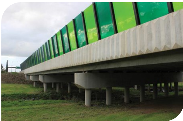
Figure 2.2. Colored panel fencing flight diverter for birds along a viaduct in Australia (Kociolek et al. 2015)
