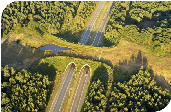
Figure 2.7. Wildlife overpass (ca. 15 m width) on concrete archway with pond in the Netherlands (Stewart 2017)
