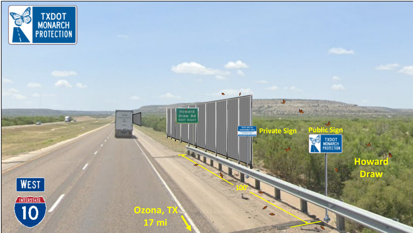
Figure 8.4. Flight diversion mesh tarp with public TxDOT Monarch Protection signage at Howard Draw Specialized Management Area #MP01.
