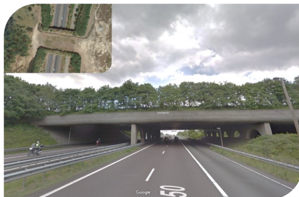
Figure 2.8. Terlet Wildlife Overpass (50 m width, 95 m length) concrete bridge span along highway A50 north of Terlet, Netherlands (Google Maps 2019)
