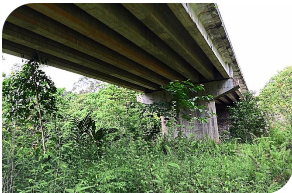
Figure 3.2. Viaduct over tropical forest in Malaysia (Li 2014)
