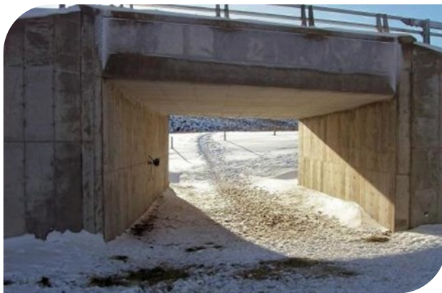
Figure 3.5. Large animal underpass box culvert (6 x 6 m, w x h) with mule deer trails along Wyoming State Highway 789, 9.7 km north of Baggs, Wyoming (Gearino 2009, Wyoming DOT 2019)
