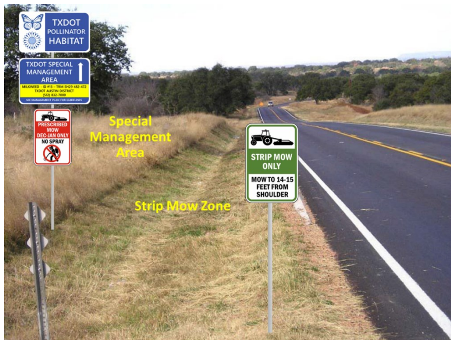
Figure 7.13. Concept for Special Management Area with strip mowing signage (background photo from TxDOT 2018a).
