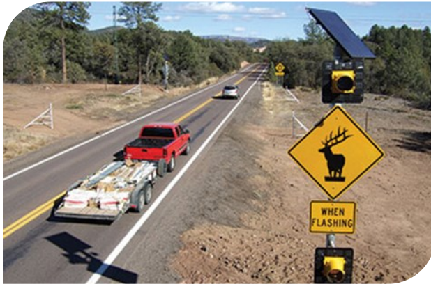
Figure 4.6. Elk crossing animal detection system wildlife warning sign with double flashing beacons near Payson, Arizona (Gray 2009)
