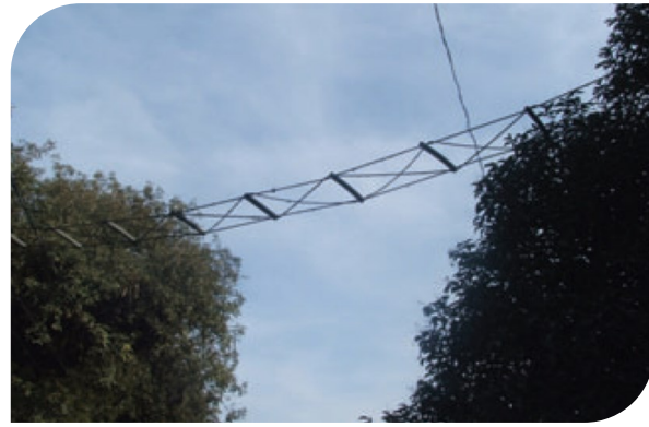
Figure 2.6. Artificial rope ladder canopy crossing used by arboreal animals in Brazil (Teixeira et al. 2013)
