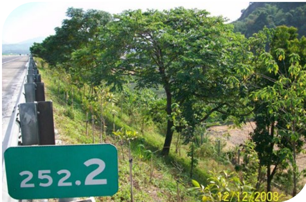
Figure 2.5. Trees planted to form vegetation screens for guiding purple crow butterfly migration above highway near National Freeway 3 viaduct near Linnei Park, Taiwan TAFNB 2008)
