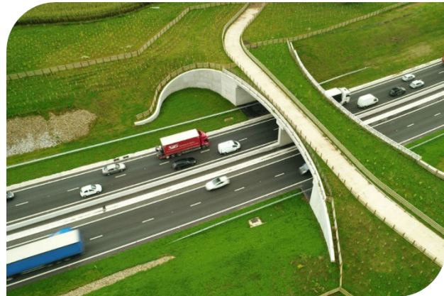
Figure 2.11. Multi-use overpass on concrete bridge span (13 m width, 65 m length) on highway A556 west of Mere, United Kingdom (Highways England 2018)
