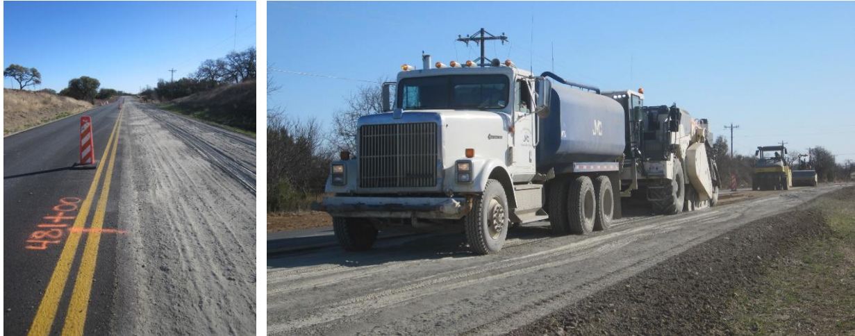
Figure 39. Cement Treatment on FM 205.
