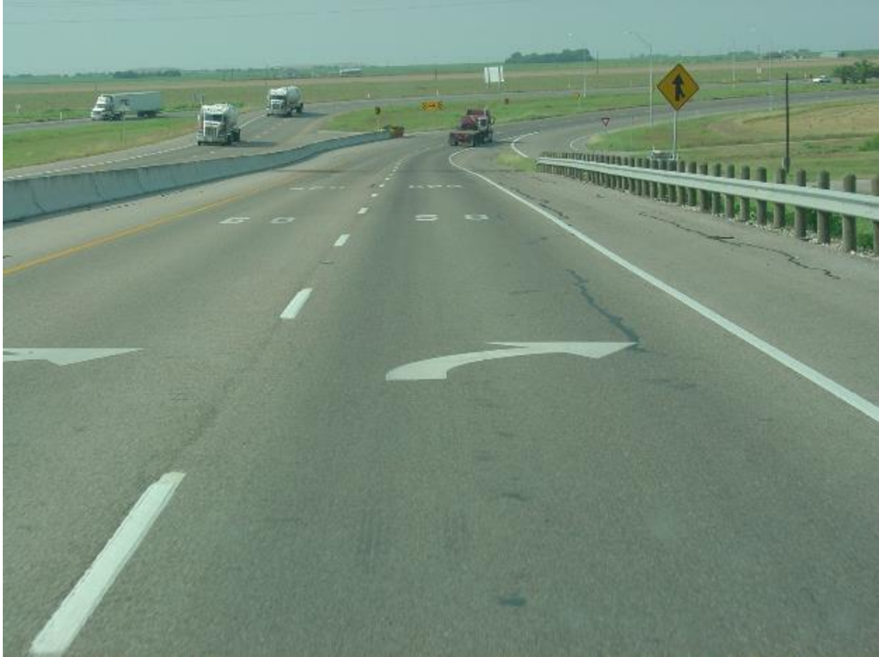
Figure 6. Urban Freeway Curve Warning Pavement Markings (7).
