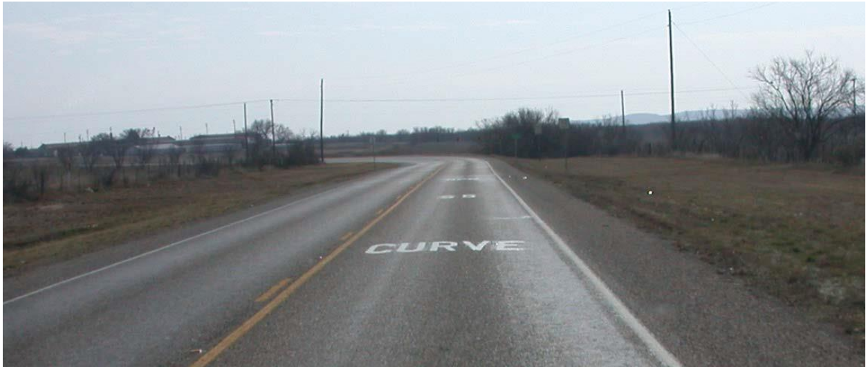
Figure 5. Text and Advisory Speed Horizontal Signing Applications (7).
