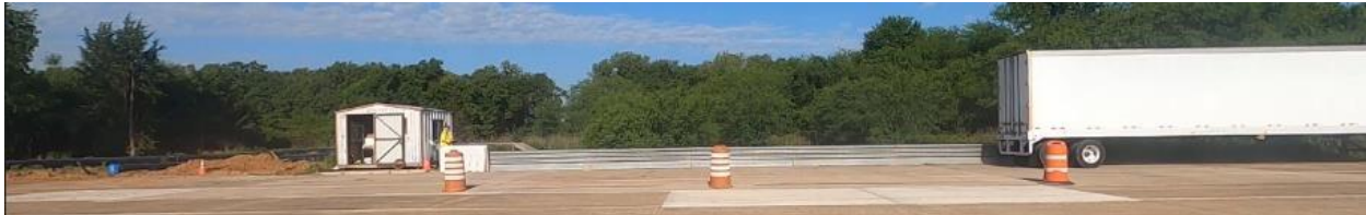
(c) Vehicle Left the RELLIS Bridge
