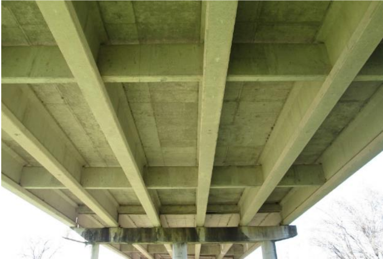
Figure 4.4: Bridge #1 Underside View.
