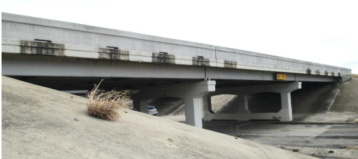
Figure 4.8: Bridge #3 Elevation View.
