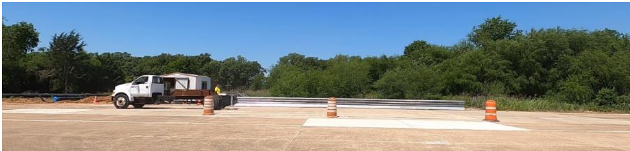
(c) Vehicle Left the RELLIS Bridge
