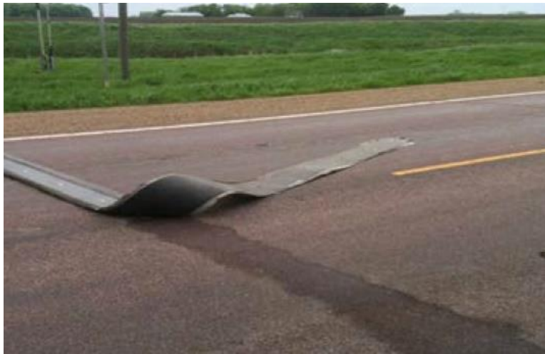
Figure 2.7. Weather-Pulled Pads (Petersen et al. 2015).
