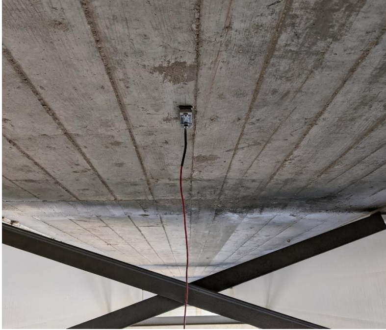
Figure 5.34. Strain Gauge Underneath the Bridge Deck (Bridge #3).
