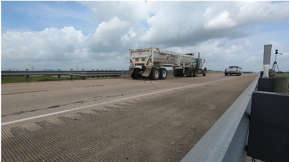
Figure 5.26. Truck Passing the Inside Lane (Bridge #2).
