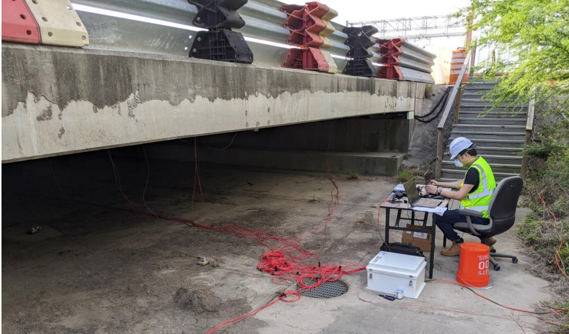
Figure 3.15. Operation of the DAQs.
