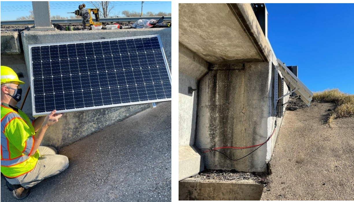
Figure 5.7. Installation of the Solar Panel.
