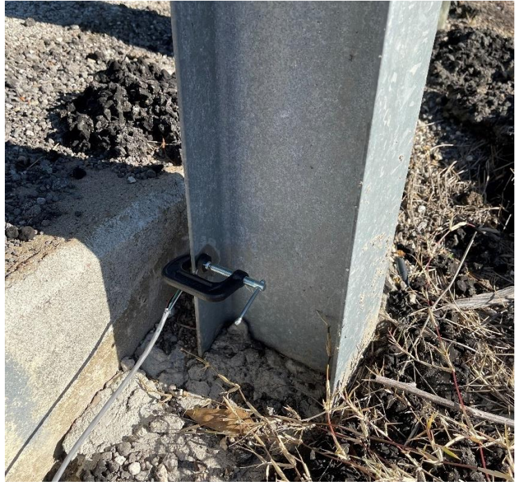
(b) Ground to the Steel Post
