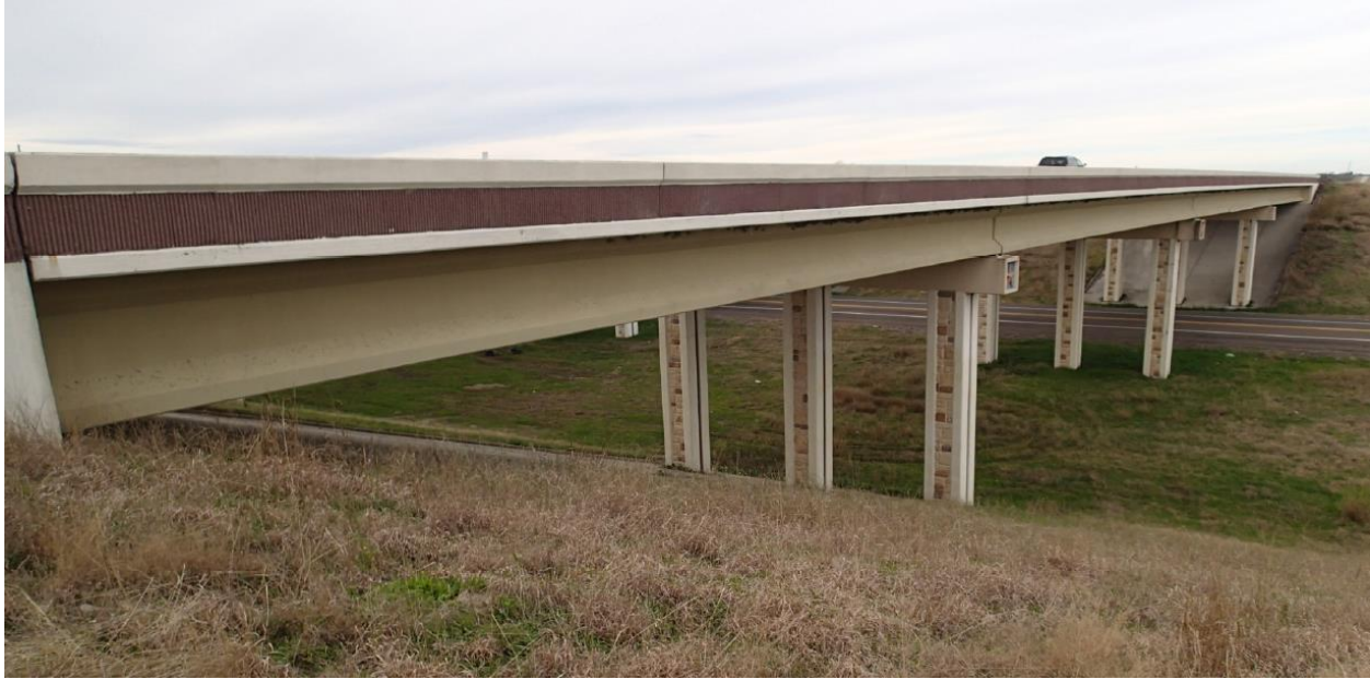
Figure 4.5: Bridge #2 Elevation View.
