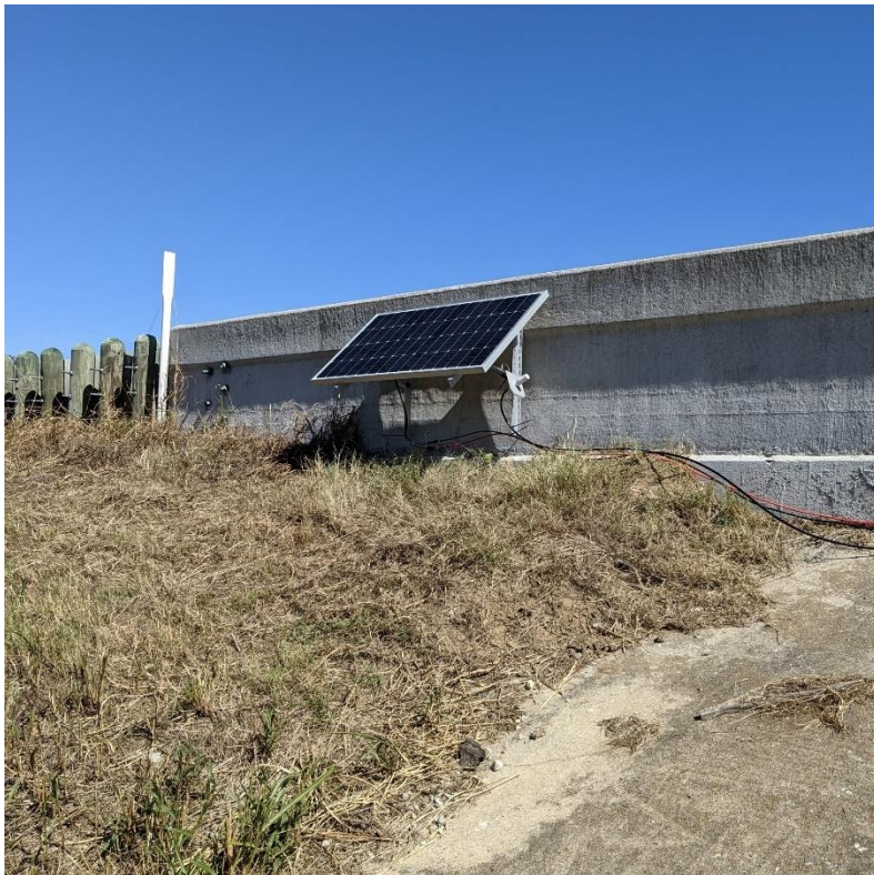
Figure 5.35. Installed Solar Panel (Bridge #3).
