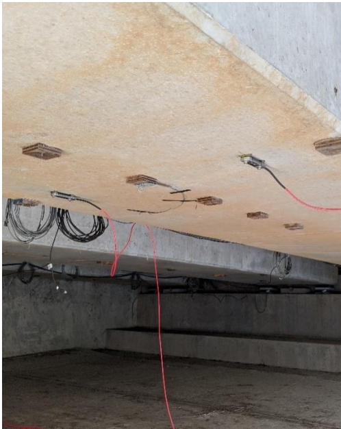
(c) Strain Gauges Installed at Midspan
