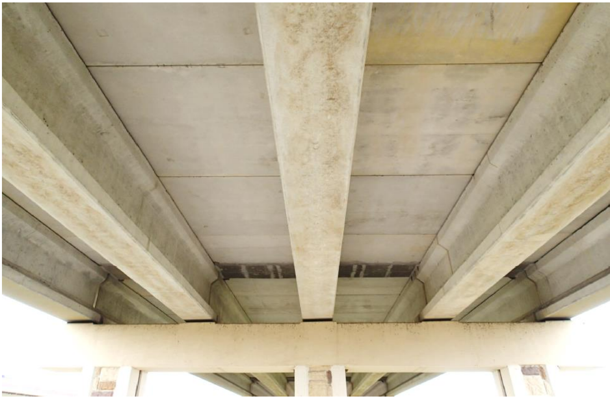
Figure 4.6: Bridge #2 Underside View.
