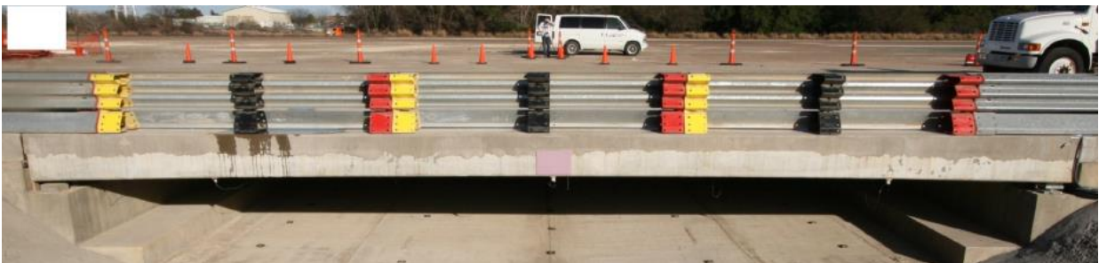
(c) Completed Bridge
