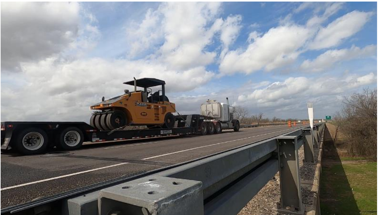
Figure 5.15. Truck B on the Inside Lane (Bridge #1).
