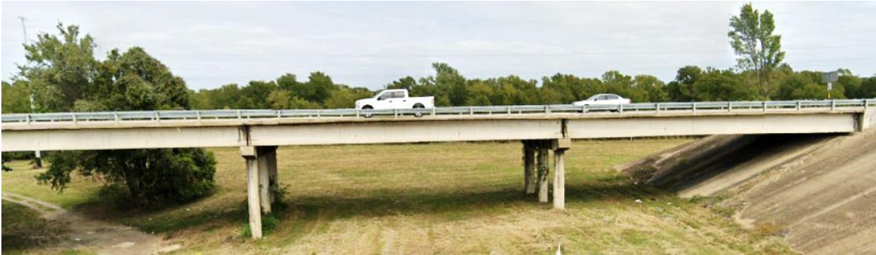
Figure 4.3. Bridge #1 Elevation View.
