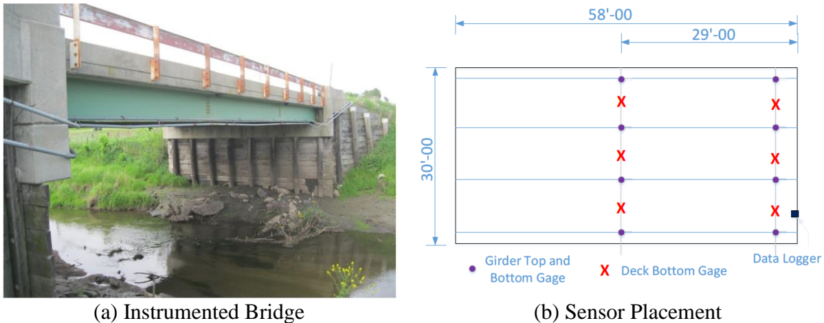
Figure 2.22. Instrumentation of the Bridge Located on Story County Road E-18 (Dahlberg et al. 2018).
