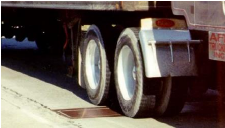
(b) Bending Plate WIM Scale Used for Vehicle Weighing ( VPG 2011 )
