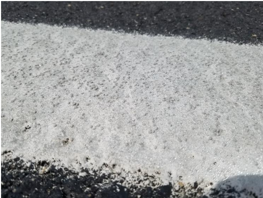
Figure 7. White All-Weather Marking with Poor Distribution of Optics.
