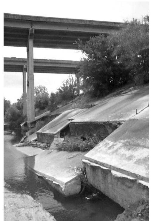
A streambank at Boggy Creek in Austin shows the effects of stream scour.
