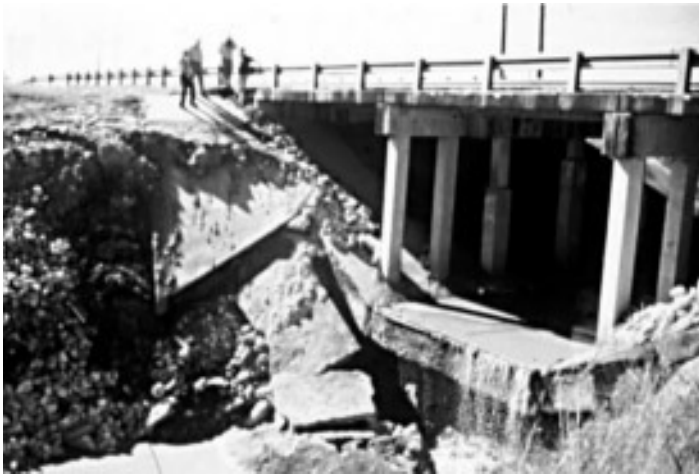
Scour — erosion of the streambed — causes serious damage to bridges every year.
