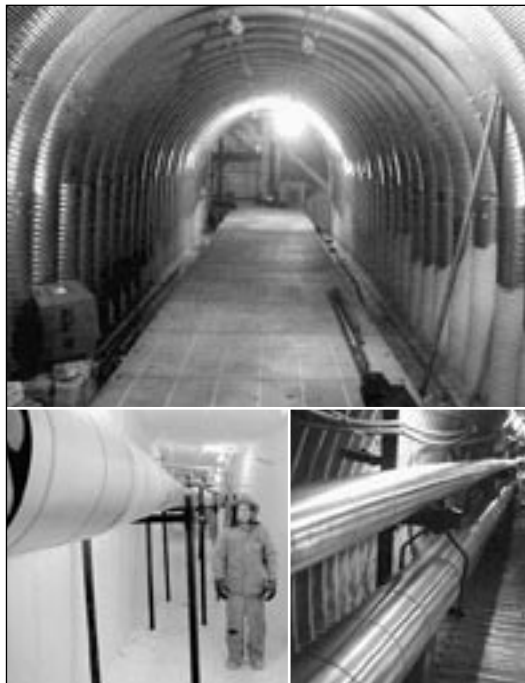
Utility corridors are being researched as one way to accommodate utilities in limited ROW space.
