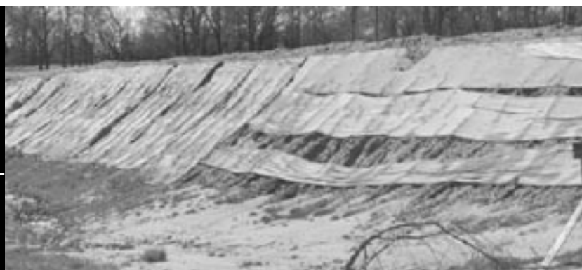
Workshop example of an improperly installed soil retention blanket.
