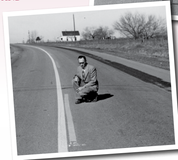
The thermoplastic pavement striper was invented at the Texas Transportation Institute (TTI) in the early 1950s. Jack Keese and his research team employed an innovative use of sulphur and heat with the paint.
