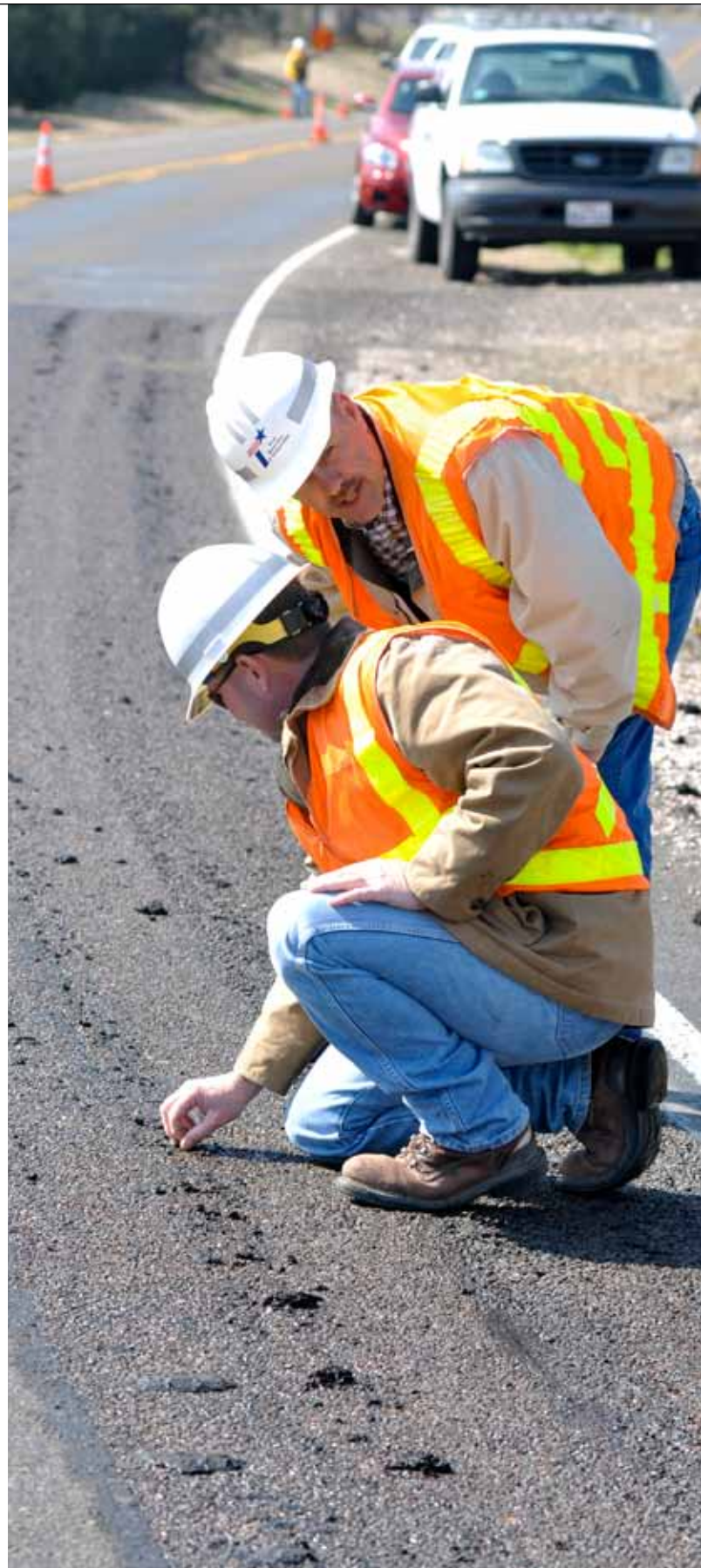
TxDOT personnel inspect the roadway after a pass from the ultra-high-pressure water truck.
