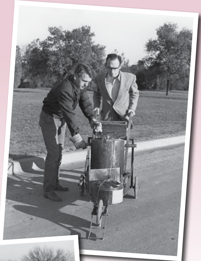
Above: A forerunner of today's automated striping machinery, the hand-powered machine was used for laying the hot-melt plastic paint stripe. It consisted of a tricycle cart, gasoline heating unit, oil-bath kettle, metal screed box (held firmly to the pavement by springs) and a wooden attachment for applying reflectorizing beads.
