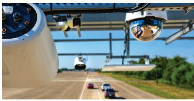
Vehicles pass through a toll gantry equipped with cameras and plate readers.
